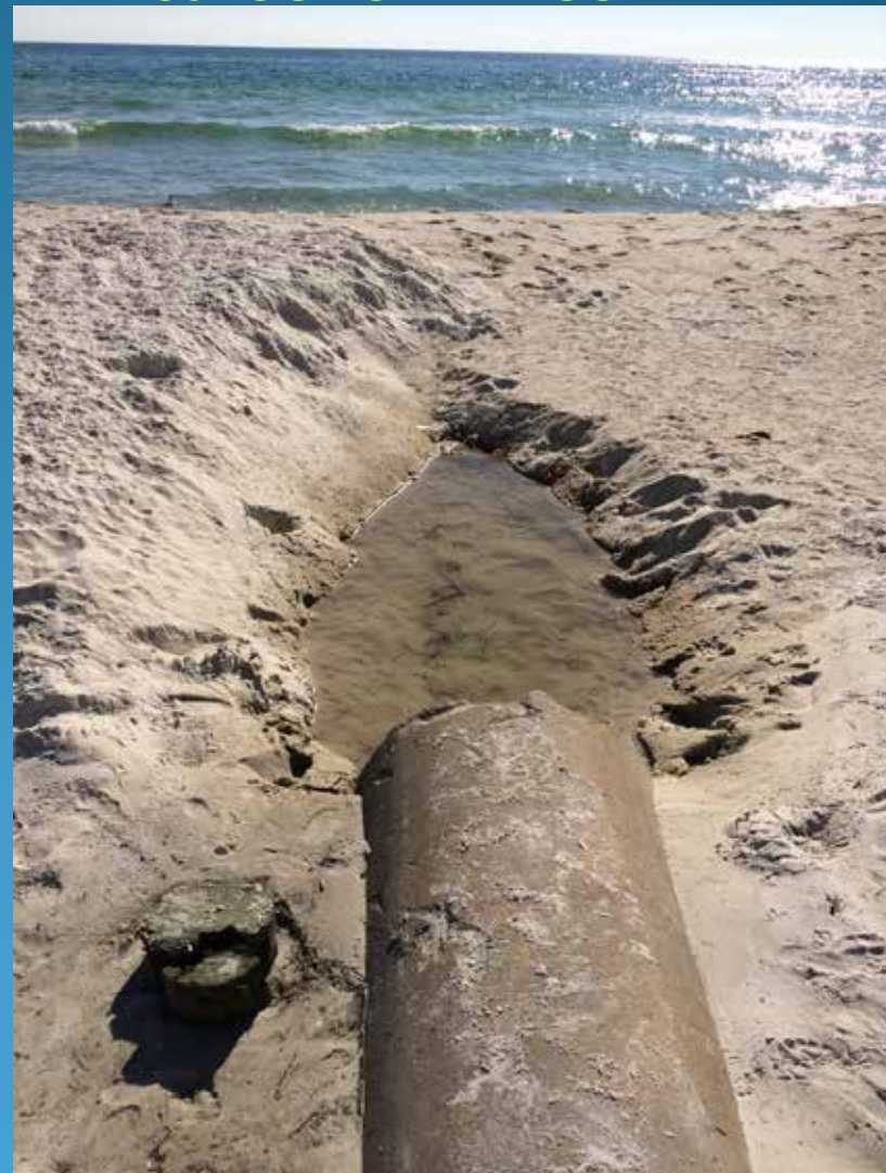
B-71 30" CONCRETE CULVERT
