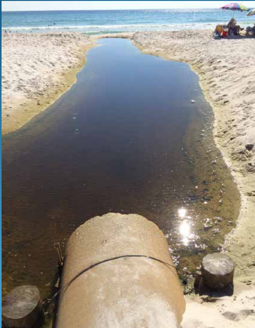
B-119 36" CONCRETE CULVERT
