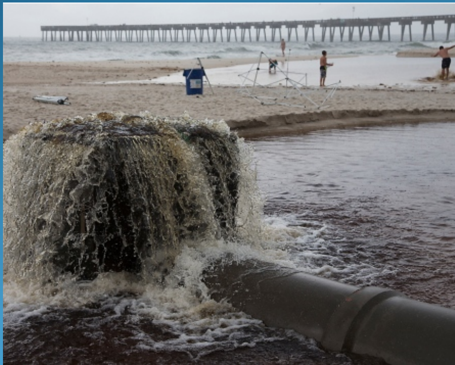
CALYPSO OUTFALL VIEW CURRENT
