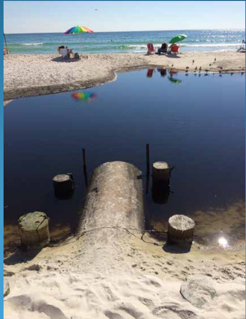
B-116 36" CONCRETE CULVERT
