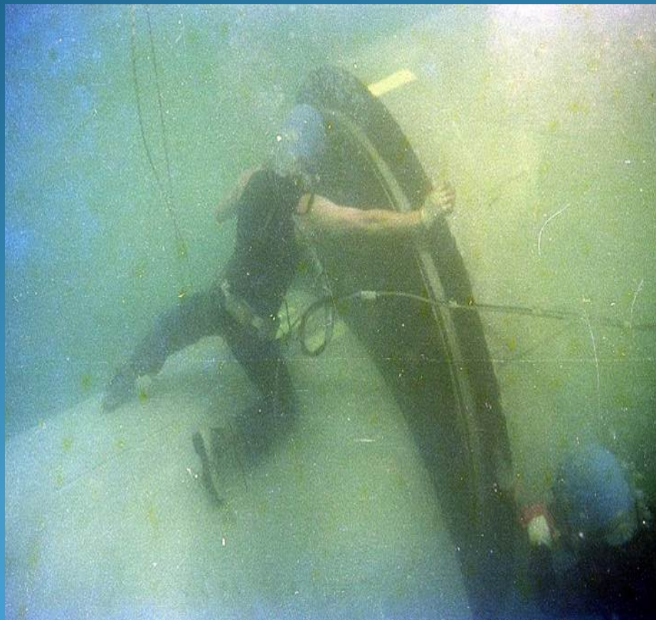
DIVER ALIGNMENT OF JOINTS
