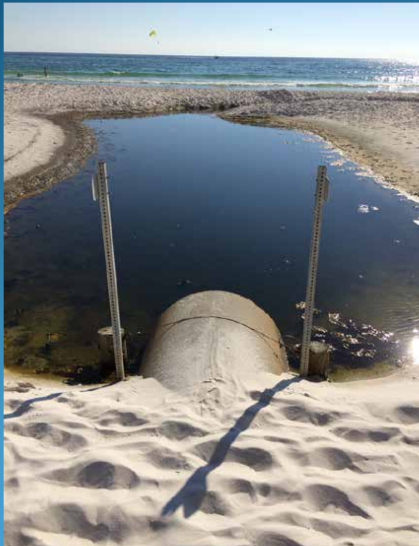
B-51 42" CONCRETE CULVERT
