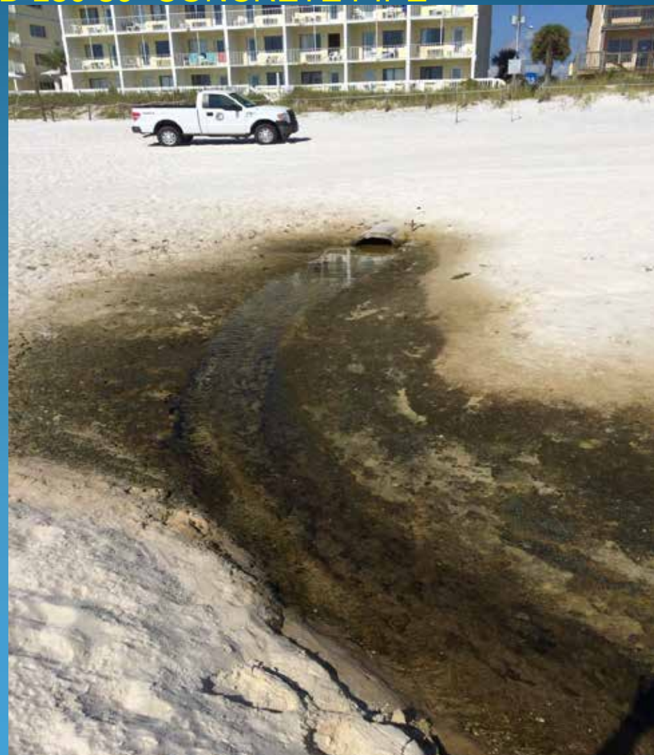
B-130 30" CONCRETE PIPE
