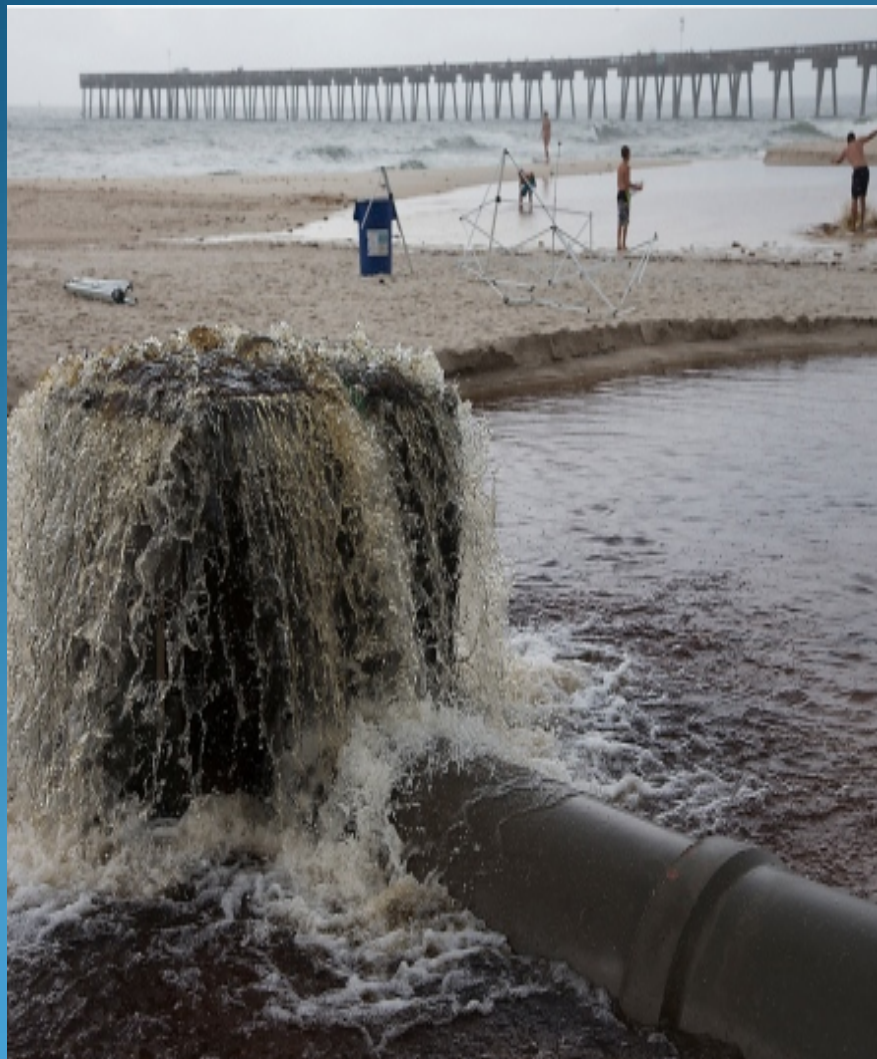
B-97 36" CONCRETE CULVERT
